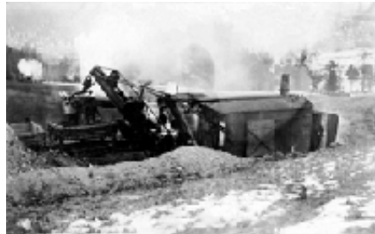
While we are not certain, the terrain suggests that the steam shovel in this view is working Clay Hill behind the Hardenburgh House in the Town of Roxbury. After leaving the cut at Clay Hill, the railroad crossed Bear Kill at Hardenburgh Falls, north of which a short tunnel was planned. (Richard F. Makse Collection)
